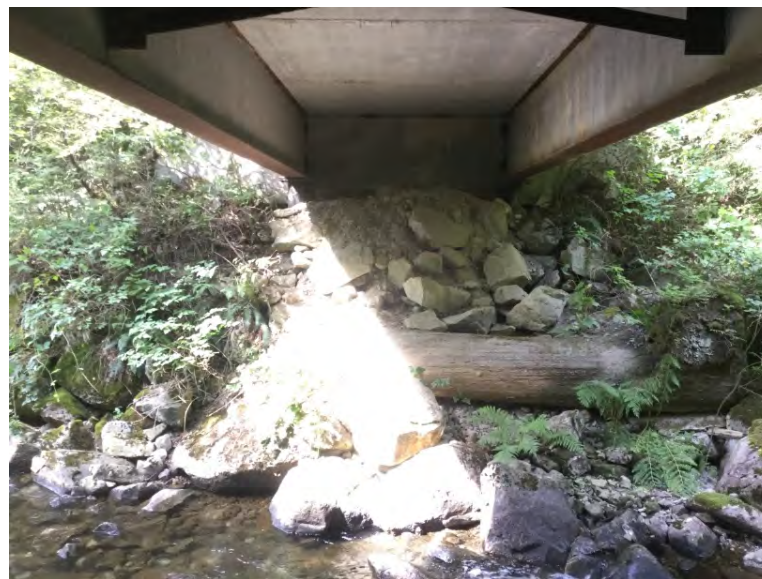
Right Bank Abutment when facing downstream
