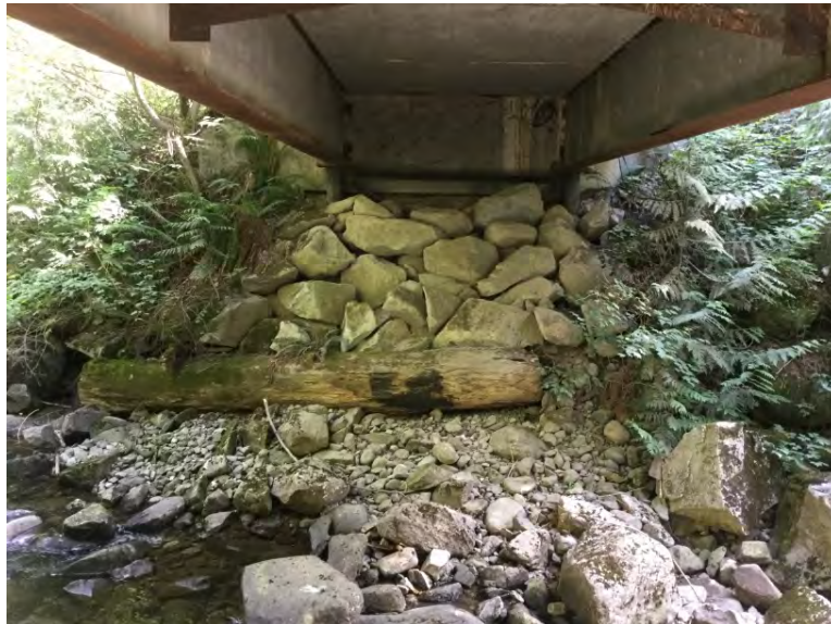
Left Bank Abutment when facing downstream
